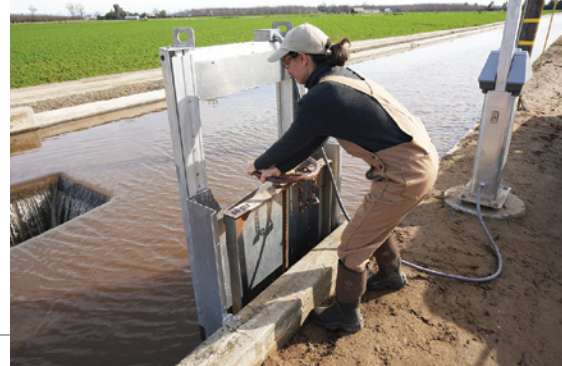
Blue Diamond grower, Christine Gemperle opens a valve to allow excess storm flows to flood a portion of her land
